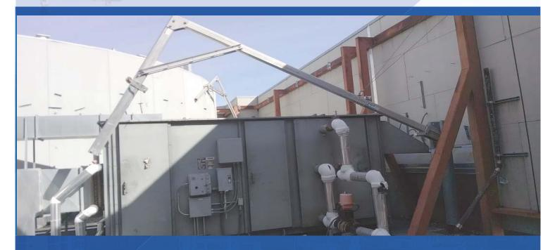
Depending on the building's features, Lynn Safety designs davits that fit the building's needs. Every project is engineered to confirm the davit system is suitable for the building
