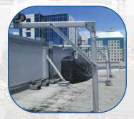
Fixed Davits are designed to remain at a fixed location as they may be either heavier than portable davits, are at an elevated location, or have a longer reach that requires they be fixed in place.
