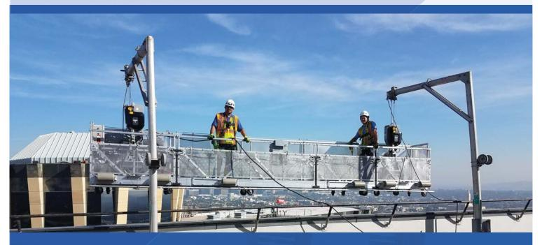
Depending on the building's features, Lynn Safety designs sockets that fit the project. Every project is designed and engineered to confirm the type of socket system selected is adequate for the building.
